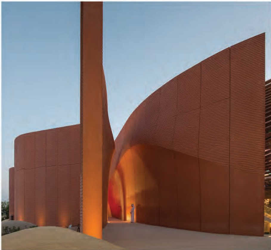
Foster + Partners, UAE Pavilion, Expo Milan The cladding material for the exterior of the drum of the UAE Pavilion and its light sources were chosen in tandem. David Atkinson Lighting Design added theatrical filters to the linear LED fixtures, specifying Tecu Gold material and a high output LED strip fitted with an amber filter
